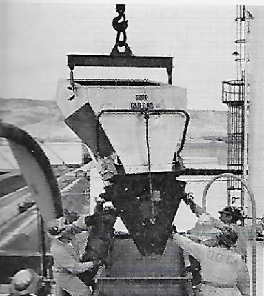
operators guide a hopper into place over a reactor, preparatory to releasing the first charge of catalyst.
